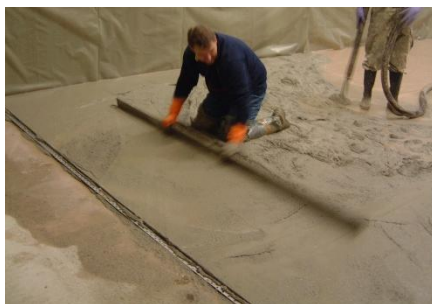
Striking off with straightedge/aluminum lath
