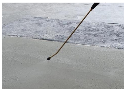
Spray EASY FINISH during trowelling process.
