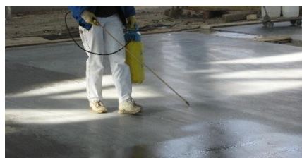
Curing with KOROMINERAL CURE
