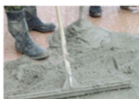
hard aggregate layer bonded on existing sub- base
