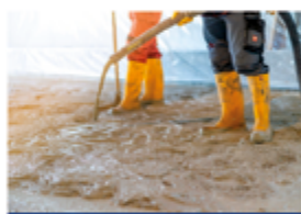
hard-aggregate layer on fresh concrete
