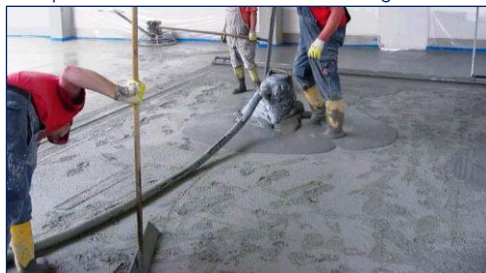
Picture 12: Striking off with leveling board / aluminum lath
