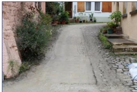
Picture 4: Grouted area, which was cleaned with high pressure water.
