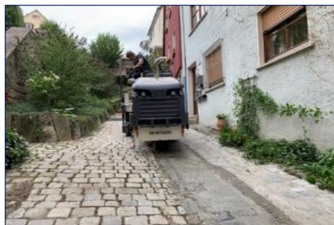
Picture 5: Milling of surface
