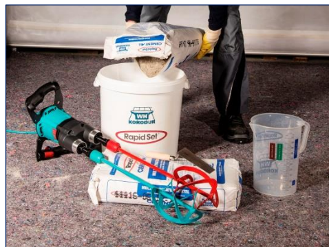
Picture 6: Mixing repair mortar for at least 3 minutes
