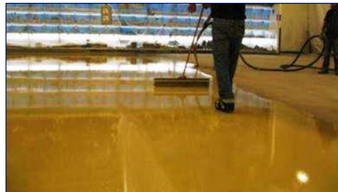
Picture 14: Polishing the surface
