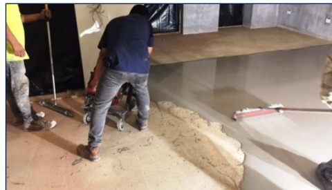
Picture 11: Application of TRU using Hippo-Mixer
