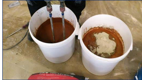
Picture 9: Admixture of colour pigments
