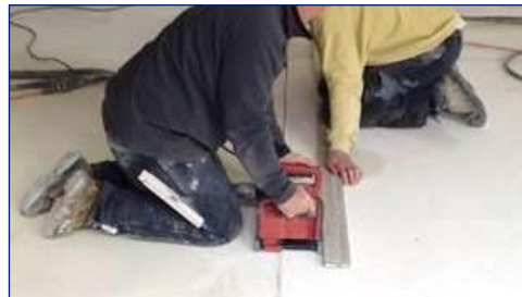
Picture 16: Application for first maintenance treatment product
