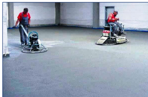
Picture 11: Smoothing with power trowel (blades) and double trowel
