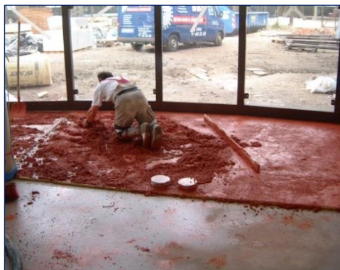
Picture 6: Grinding/floating the surface
