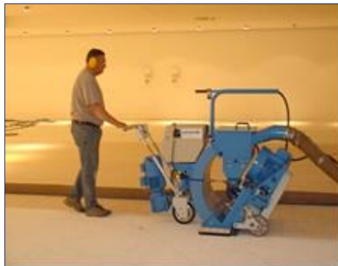
Picture 2: Thorough pre-wetting of the clean sub-base, avoiding puddle formation
