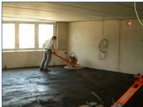
Picture 7: Troweling of surface
