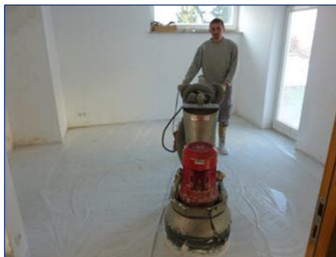
Picture 14: Application of first maintenance product
