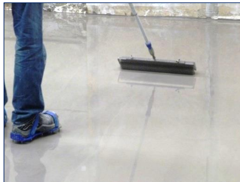
Picture 11: Spiked roller for venting
