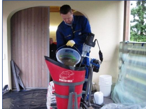
Picture 8: Application with hand mixed NEODUR Level
