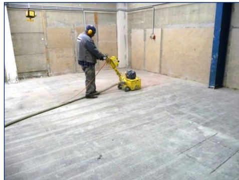
Picture 1: Preparing the surface by milling
