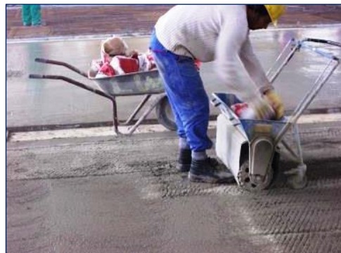
Picture 4: Dry-shake application with spreader
