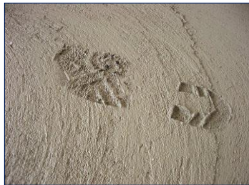
Picture 2: Troweling (disk) of surface
