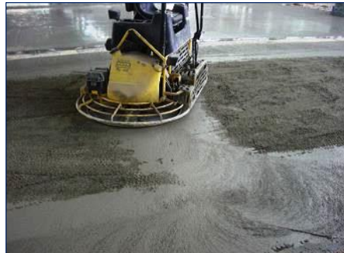
Picture 8: Troweling of surface using double trowel
