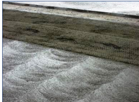
Picture 6: dry-shake application with spreader
