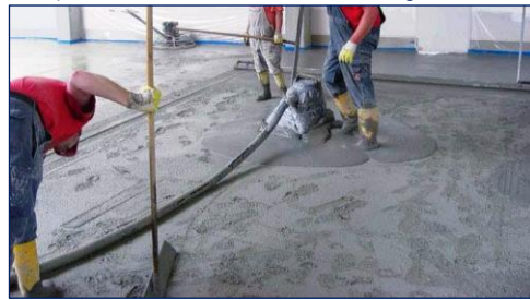
Picture 12: Striking off with leveling board / aluminum lath
