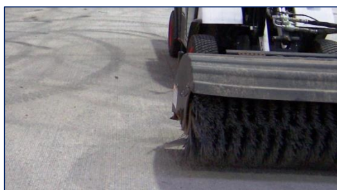
Picture 4: Pre-wetting of sub-base matt-damp
