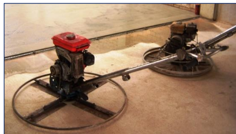
Picture 16: Power trowel (blade and doublet trowel in work
