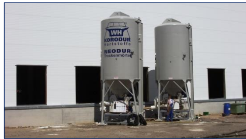
Picture 10: Material application with feeding hose
