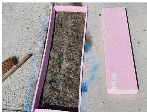
Picture 7: Preparation with edging strips
