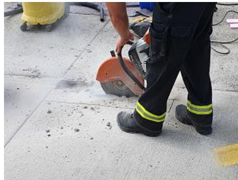
Picture 1: Cutting the affected part of the slab
