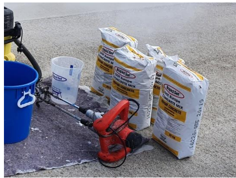
Picture 4: Dose mixing water in 5-liter measuring cup and pour into the mixing container
