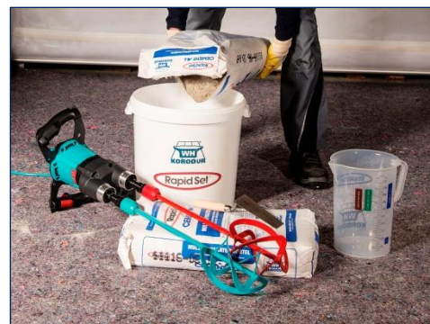
Picture 6: Mix repair mortar for at least 3 minutes
