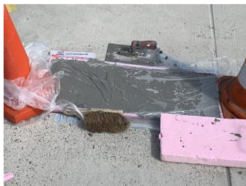
Picture 11: Curing the finished area for at least 1 hour
