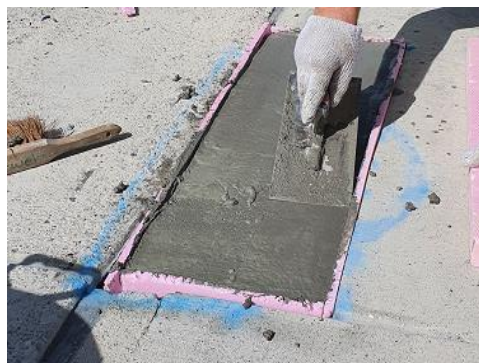
Picture 10: Smoothed concrete surface
