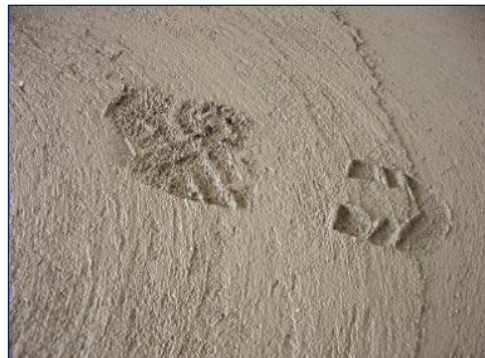
Picture 2: Troweling (with disk) the base concrete
