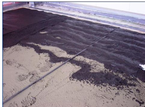
Picture 8: Application of the hard aggregate floor “fresh on fresh” using round bars (leveling gauges)
