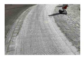
To improve the traffic safety in a roundabout in Göppingen, a paved lane was renovated on basis of a **special procedure** developed by Blessing and KORODUR, based on **Rapid Set Mortar Mix**. Read more
