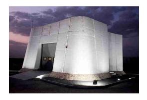
We are proud that the DEWA's Robotics and Drone laboratory (DEWA = Dubai Electricity and Water Authority), which was produced with our partner CyBe Construction using 3D Concrete Printing, was included in the Guinness Book of Word Records 5 years after completion (including building permit)! Read more.
