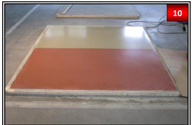
The drying time up to foot traffic is usually about 7 hours, but may vary depending on ambient temperature, humidity and material consumption. Do not strain or cover the treated surface for 48-72 hours. Moreover, it should not be driven with floor scrubbing machines during that time.
