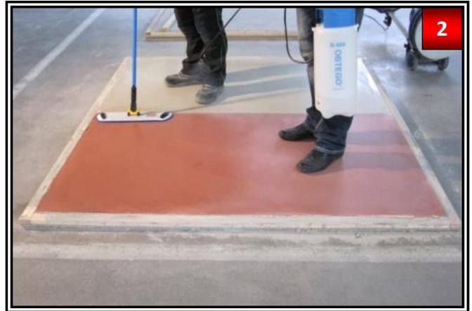
Apply OBTEGO® R-400 homogenously with a pump sprayer and work the product into the floor with a microfiber mop. Recommended fan nozzle 0,1.
