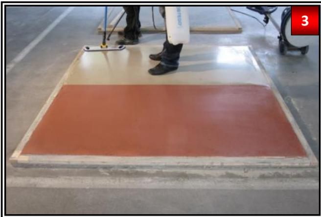
Consumption of the material during first application is approx. 40-50 ml/m<sup>2</sup>. The application is done in tracks. The track width follows automatically trough the wiper (approx. 1 m).
