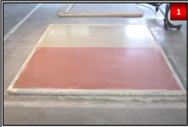
TRU self-leveling floor grinded with diamond grinding machine and polished up to 800 grit (sample application). Before application, surface must be dust free and dry. (\*1)
