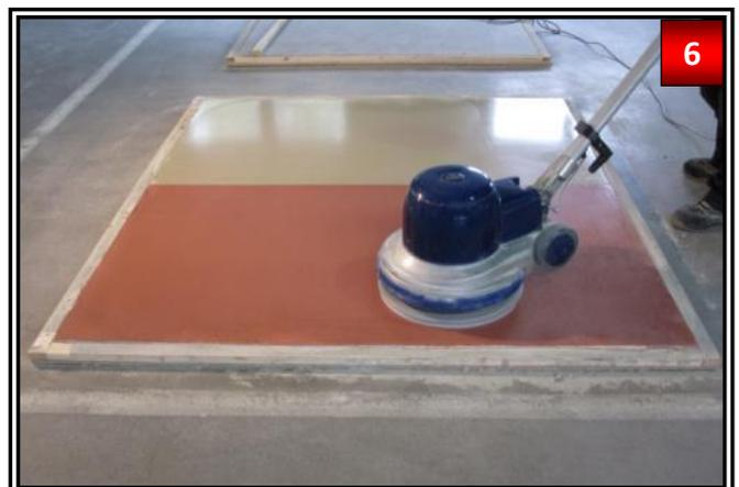
Before the material dries up (depending on temperature and humidity between 2 – 10 min.), buff the oily smear film with a single disc machine and a white polishing pad into the floor.
