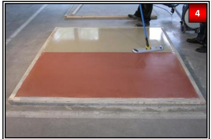
The floor must be saturated with R-400, but there should be no thick excess material onto the floor. Avoid excess material onto the surface even in overlapping areas.
