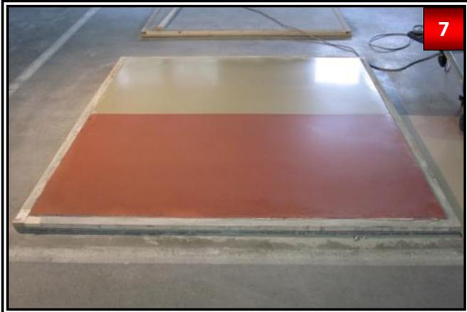
Allow OBTEGO® R-400 to dry 1-2 hours, if possible better over night. The floor absorbs the product further, which makes a second application necessary.
