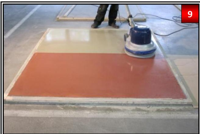
During buffing pay attention to uniform appearance. Avoid large excess material, splashes and marks from the buffing machine. The pad becomes sticky and the surface slightly matt, if buffed too long with the machine on the same area.
