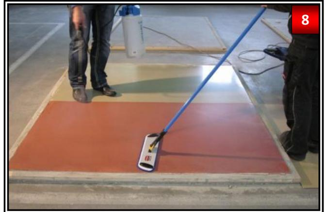
Second application of OBTEGO® R-400 is made as step 2-6, but carried out crosswise to first application. Material consumption during second application approx. 20-30 ml/m².
