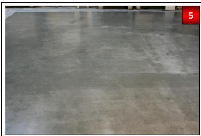
Because of different absorption of some floors it could come to different drying up of OBTEGO® P-20 pore filler. The curing time amounts between 1-2 hours.
