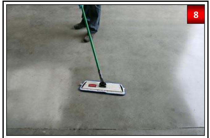
When wiping, make sure that all surfaces are achieved with the product. On the surface, should be remain a thin, slightly greasy film.
