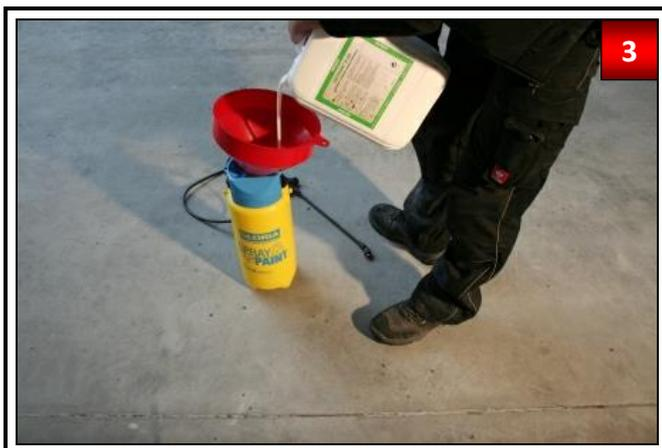
Fill in OBTEGO® P-20 pore filler in spray pump and put containers under pressure. For a good spraying result we recommend airless nozzle 0.25 / 80 °.
