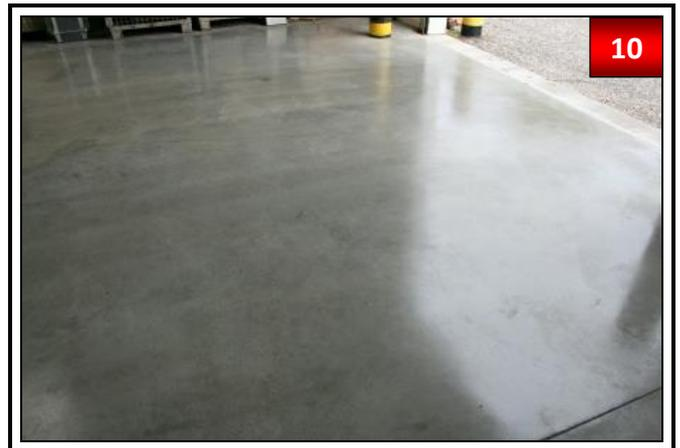
Don't use heavy equipment such as fork lifter until complete cure (24-48 hours). It should also not be operated with auto scrubber within this curing time.
