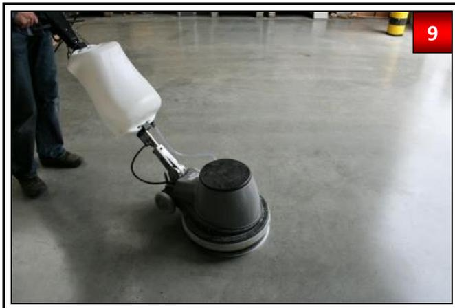
Shortly after wiping with the mop, use a white polishing pad and polish over the surface. Don't enter into the polished surface before the film is completely dried. The drying time is usually about 6-7 hours, but may vary depending on ambient temperature and floor surface.
