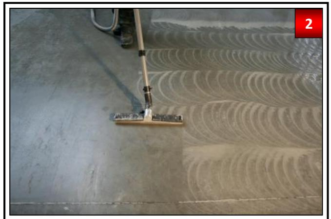
Then soak up and repeat process 1-2 with clear water to neutralize the floor.
