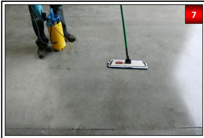
Apply OBTEGO® R-400 uniformly by spraying on the surface and distribute additional with microfiber mop. We recommend to use microfiber mop which are used for waxing.
