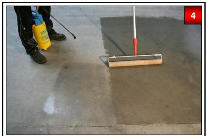
Apply OBTEGO® P-20 pore filler uniformly on the surface and use roller immediately (e.g. nylon roller, 5-8mm) to achieve a homogeneous appearance.
