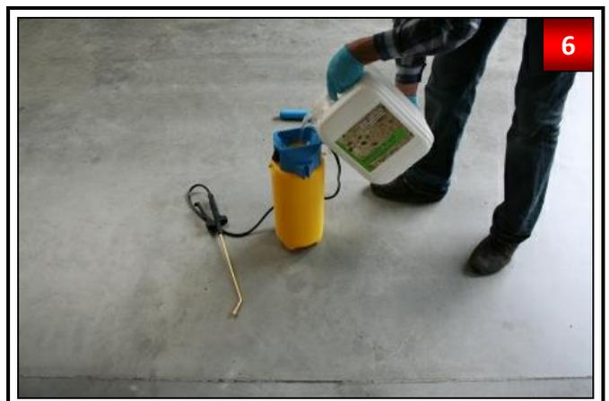
After completely drying up of P-20, fill in OBTEGO® R-400 in a separate spray pump and put container under pressure. Standard nozzle for fine spraying is recommended.
